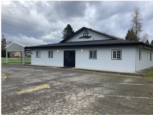
MW Roof & Ext Paint
