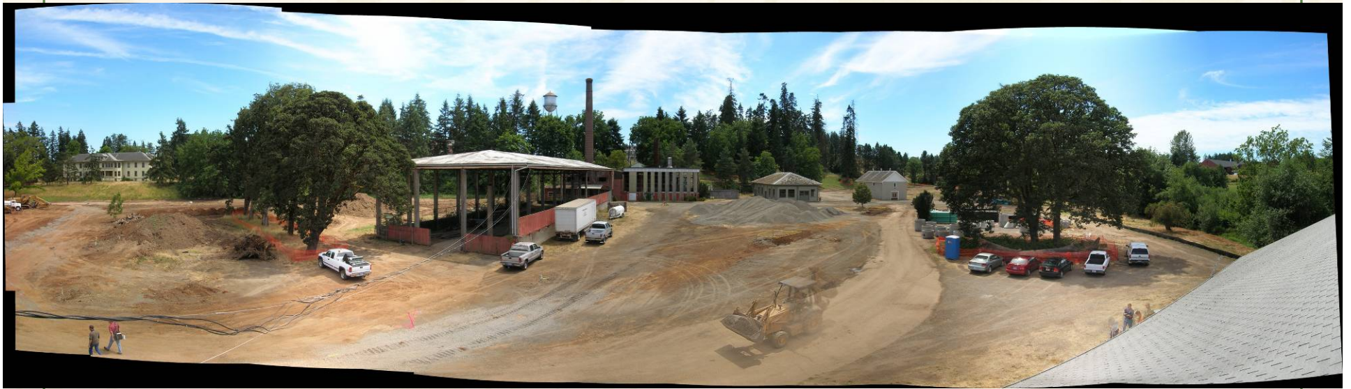
Construction staging in the Village Center.
