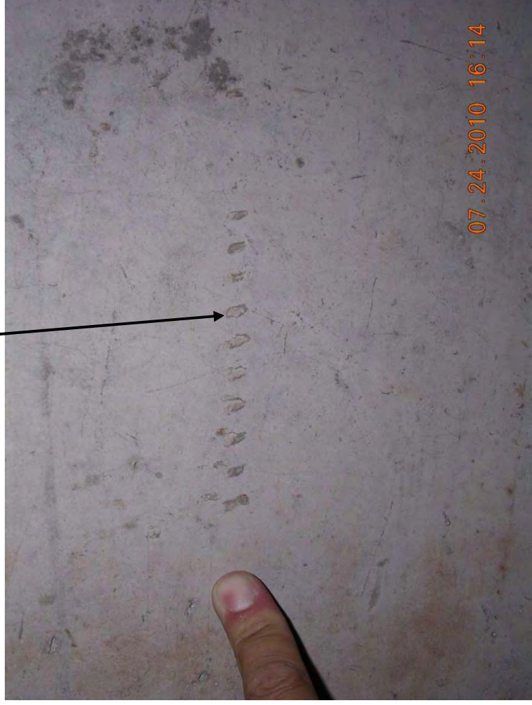
REINFORCING BAR EXPOSED AT THE BOTTOM OF THE BUS MALL SLAB
