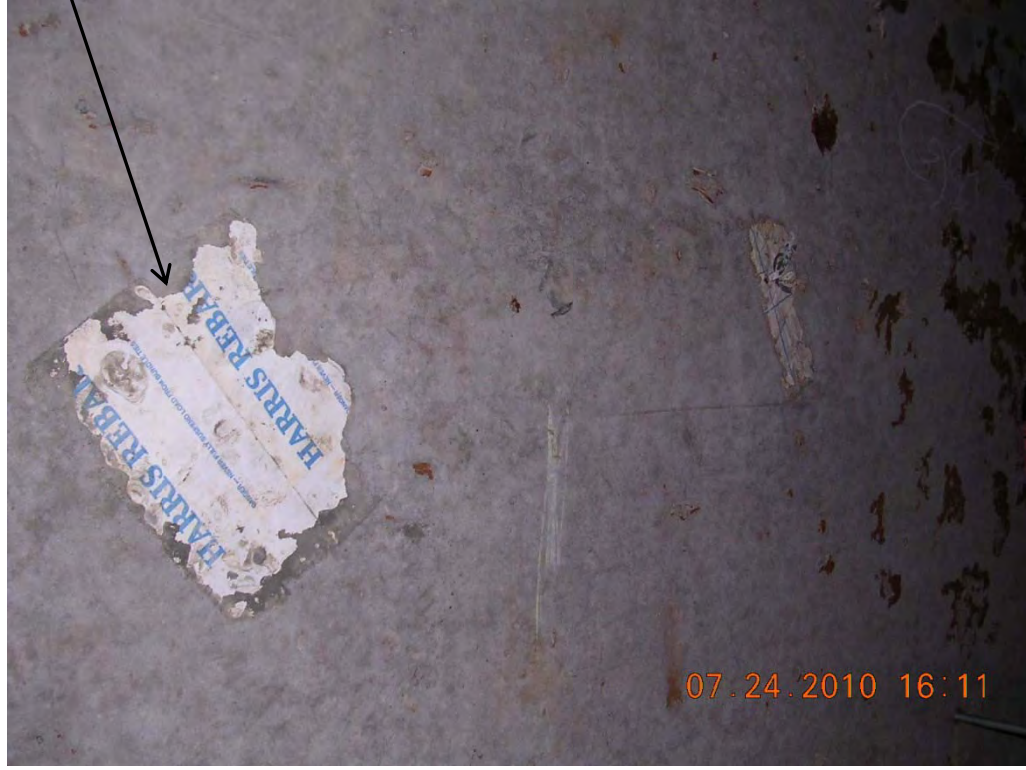
Debris on the form work cast into the Bus Mall slab.
