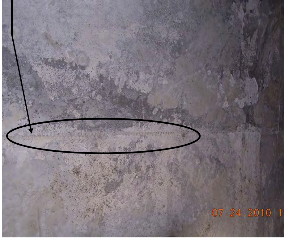
REINFORCING BAR EXPOSED AT THE BOTTOM OF THE BUS MALL SLAB
