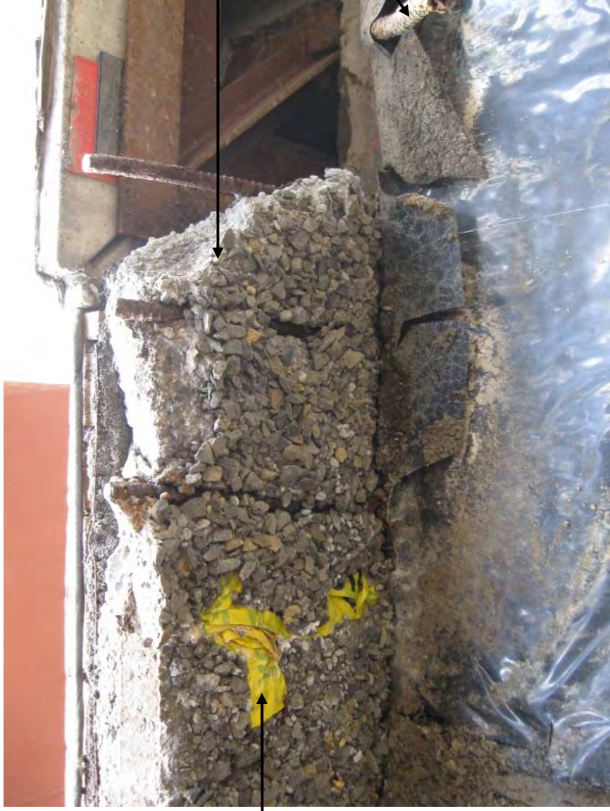
DEBRIS IN CASTING BED
