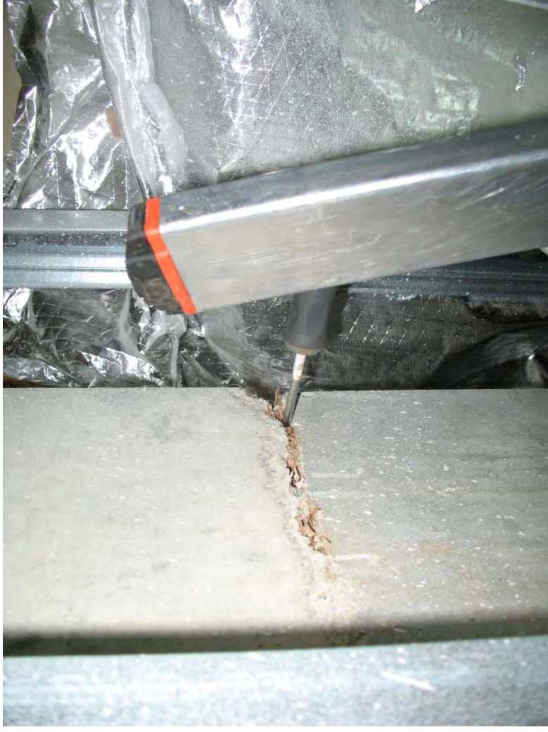
Wood Chips Cast Into Concrete Column
