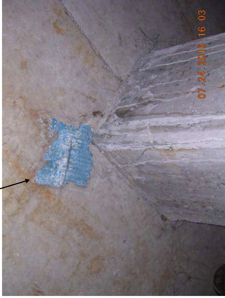
DEBRIS ON THE FORM WORK CAST INTO THE BUS MALL SLAB
