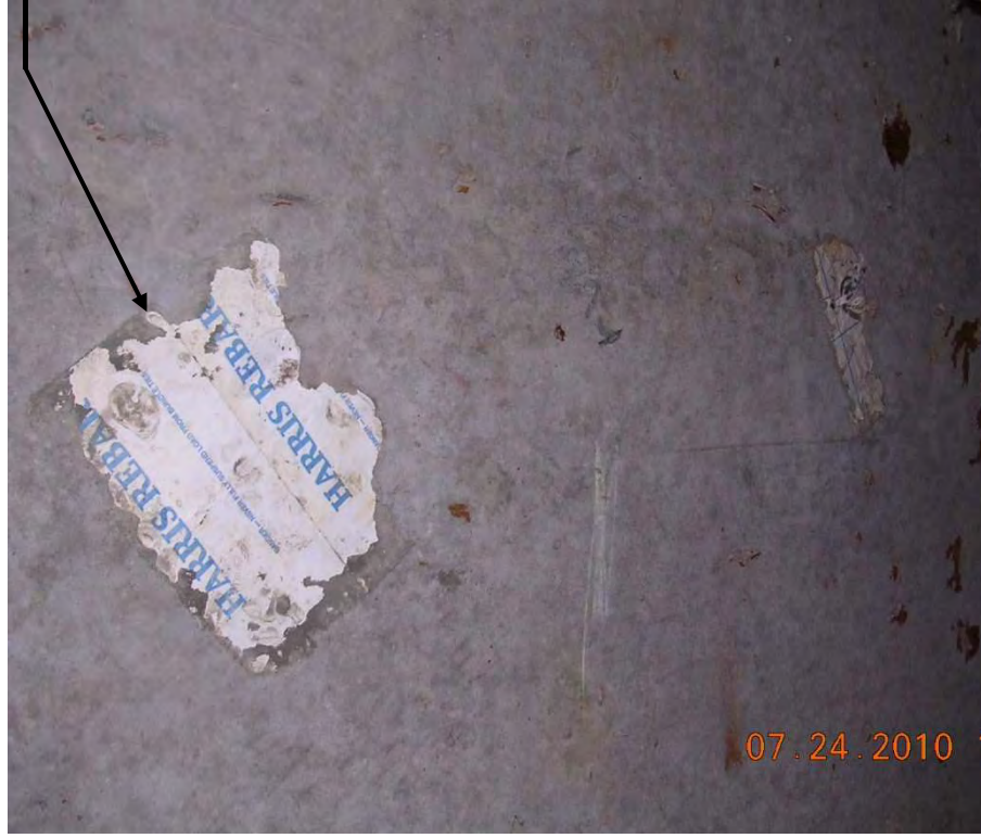
DEBRIS ON THE FORM WORK CAST INTO THE BUS MALL SLAB
