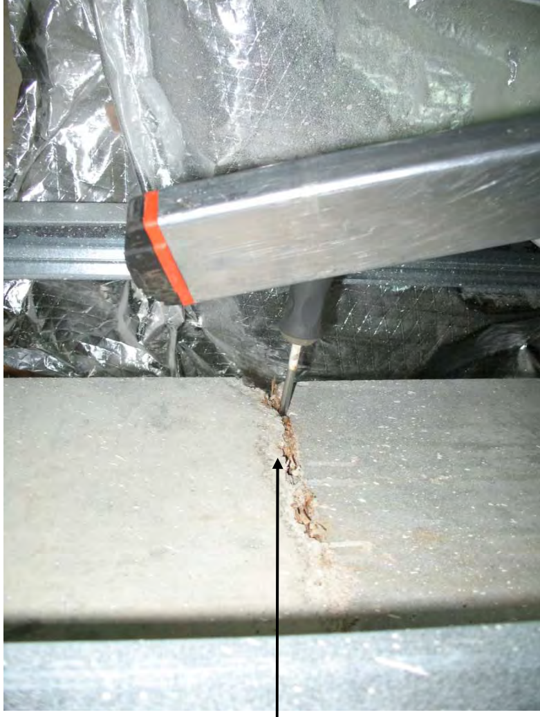
Wood Chips Cast Into Concrete Column
