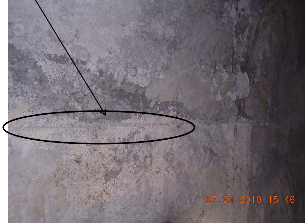
Reinforcing bar exposed at the bottom of the Bus Mall slab.
