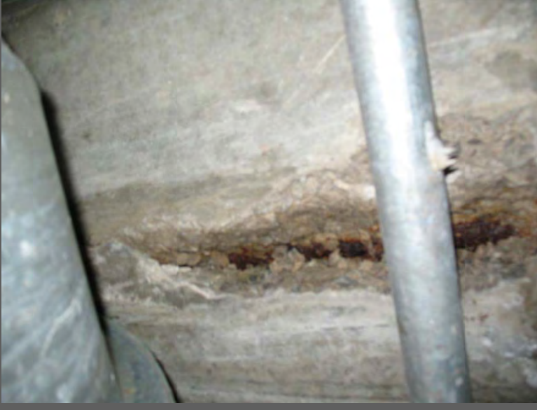
Crack w/spall removed at Grid O-10
