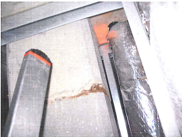
Wood fibers cast into the concrete column Date: April 14, 2010
