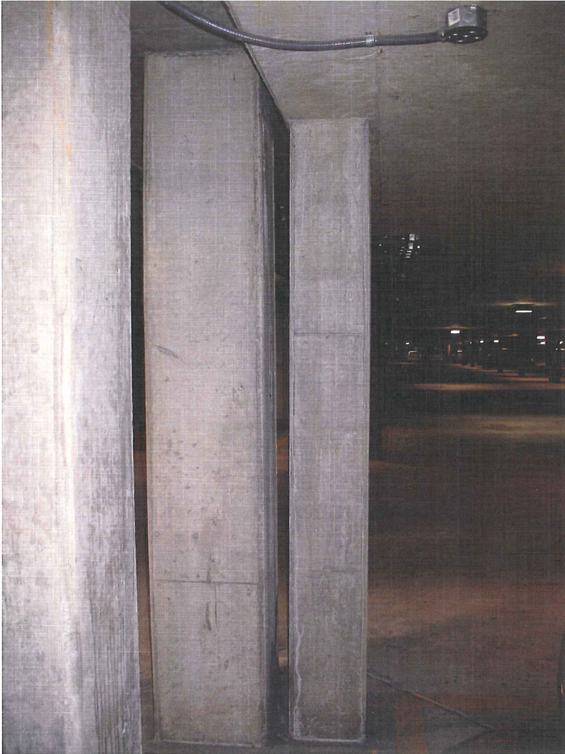
Between Marion County Courthouse Building and Bus Mall Column leans to the North 1\frac{1}{2} " at the top along Gridline 10 Date: April 14, 2010
