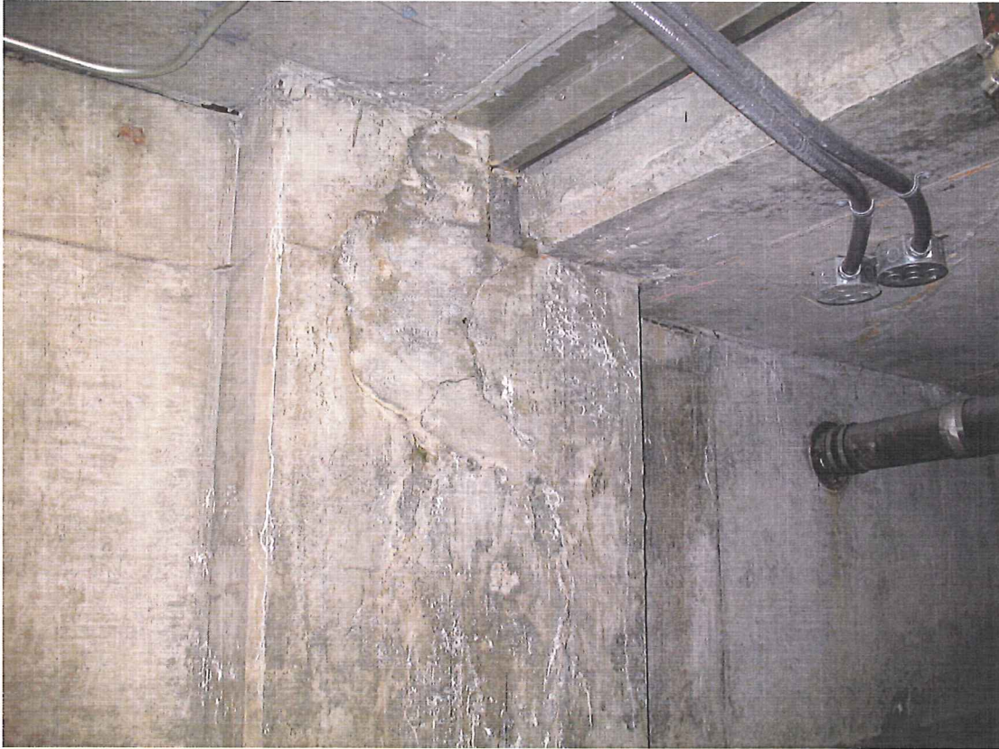
Significant cracking at the expansion joint between Bus Mall and North Block (Grid O-3a) Date: April 14, 2010
