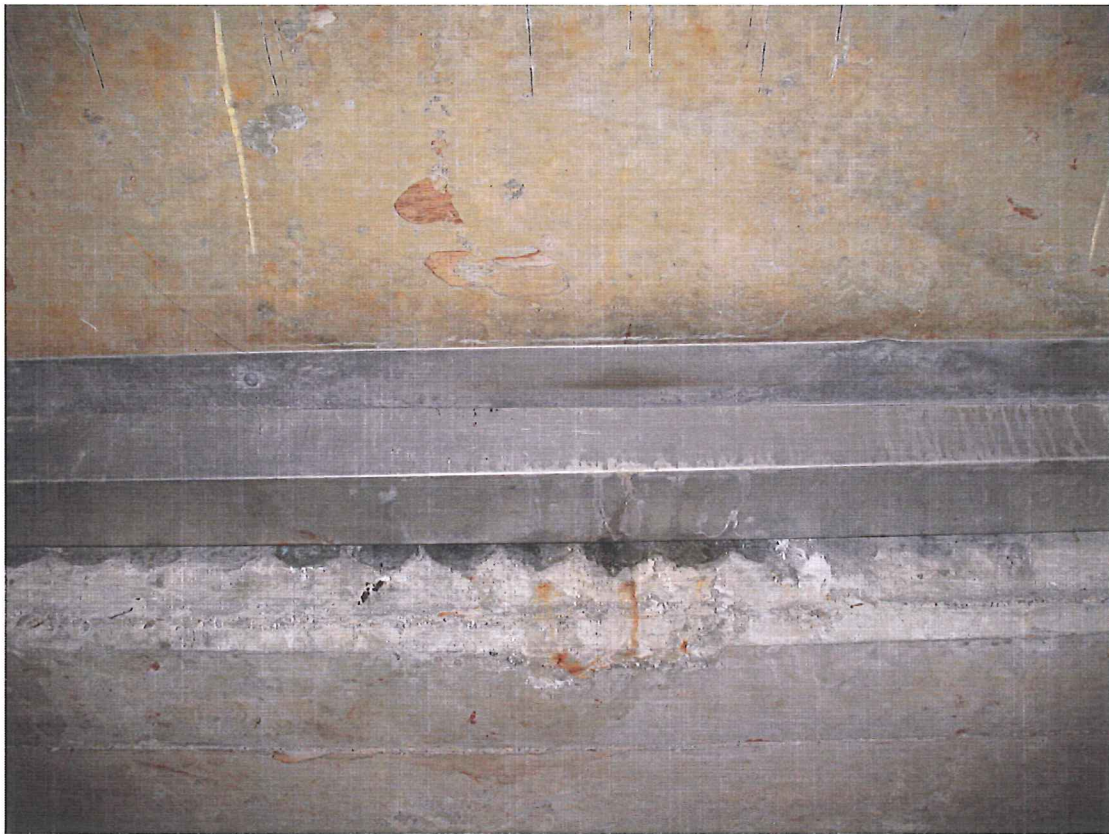
Tendon grout pockets with spalling of the grout pockets visible as a result of moisture penetration North edge of the bus mall slab Date: April 14, 2010
