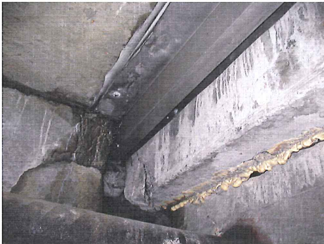
Significant cracking at the expansion joint between the Bus Mall and the North Block Date: December 1, 2010
