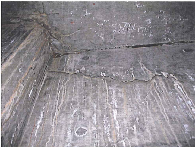
Significant cracking and efflorescence coming through concrete at Northeast corner column (Grid N1-1) Date: April 14, 2010
