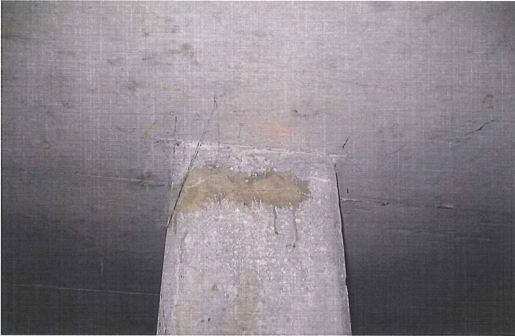
Grid B-9: Visible construction patch with typical cracking (0.20 mm)
