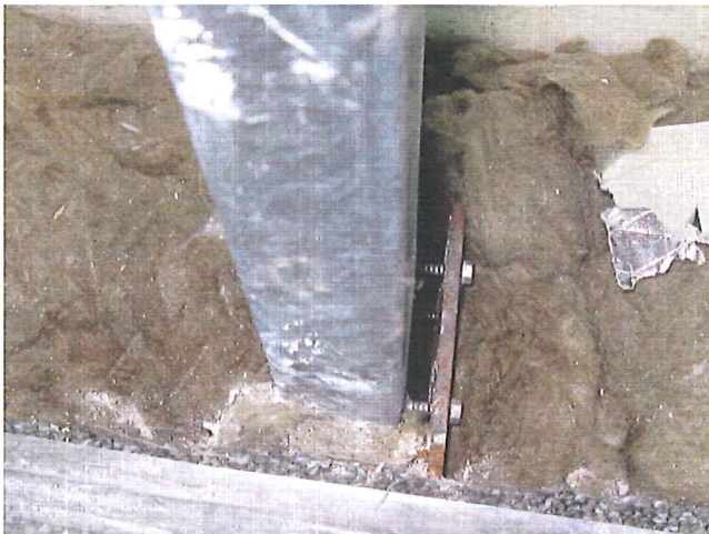
Separation between the exterior structural light gauge steel stud and connection plate Date: June 3, 2010
