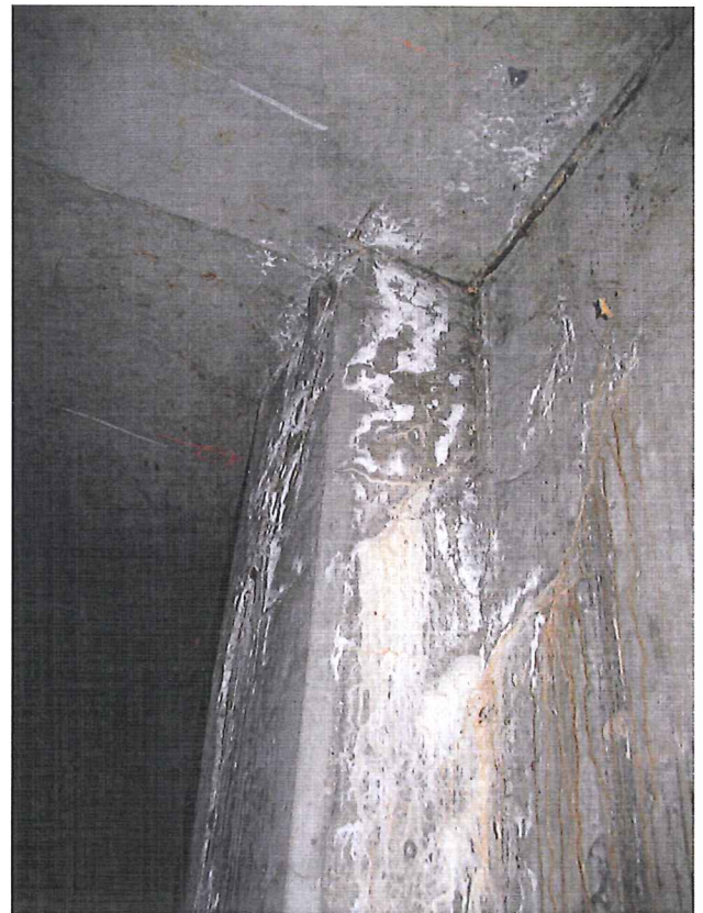
Significant cracking and efflorescence coming through Concrete column at Grid M-1 Date: April 14, 2010
