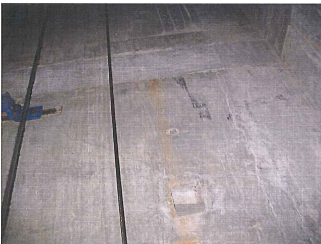
Elevator Hoistway – Diagonal crack near a floor slab Date: April 14, 2010
