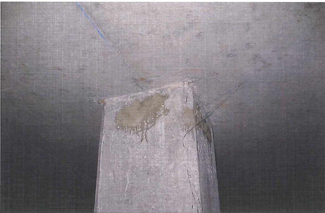
Grid B-9: Visible construction patch with typical cracking (0.20 mm)
