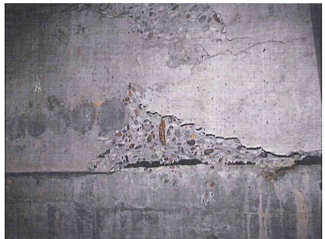
Cracking of the Bus Mall slab edge visible from the North Block along Gridline 3a Date: December 1, 2010
