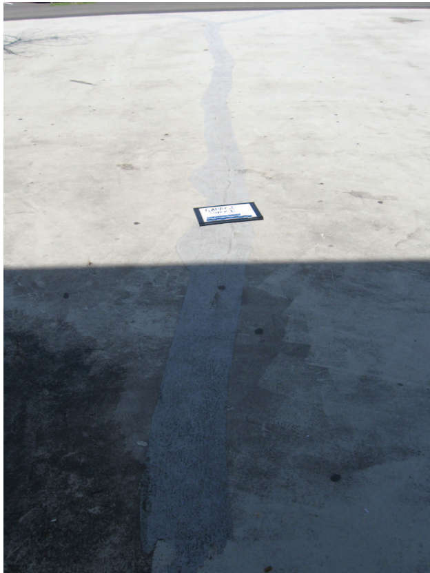
All photos: Cracks at the North Block slab.
