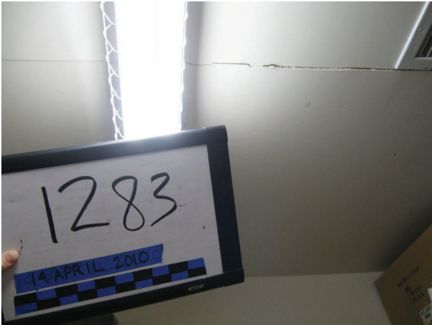
Top left: Ceiling crack in a utility space.
