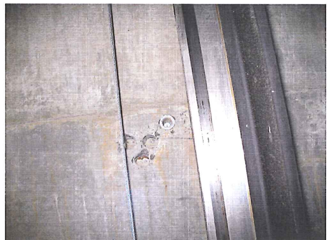
Elevator Hoistway – Installation of a drop-in anchor (Reinforcement is visible as a result of previous anchor installation attempts) Date: April 14, 2010
