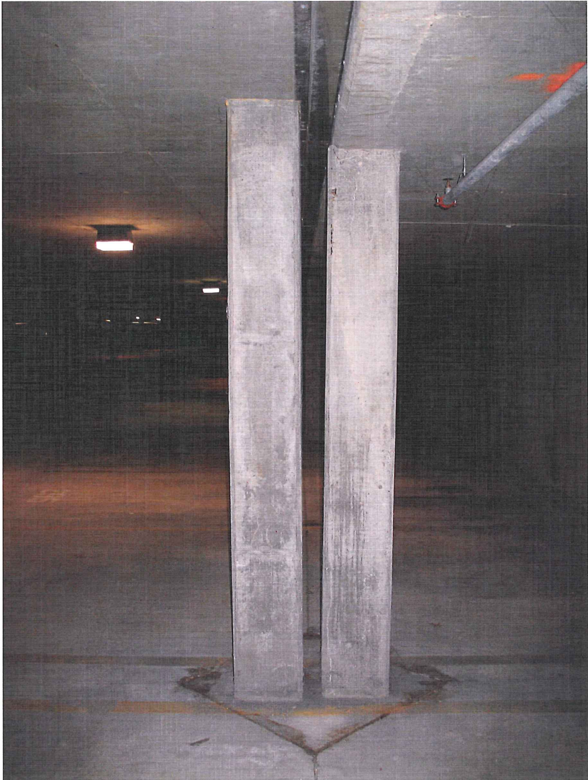
Between Marion County Courthouse Building and Bus Mall (Grid E-3a) Column leans to the South 1½" at the top along Gridline 3a Date: April 14, 2010
