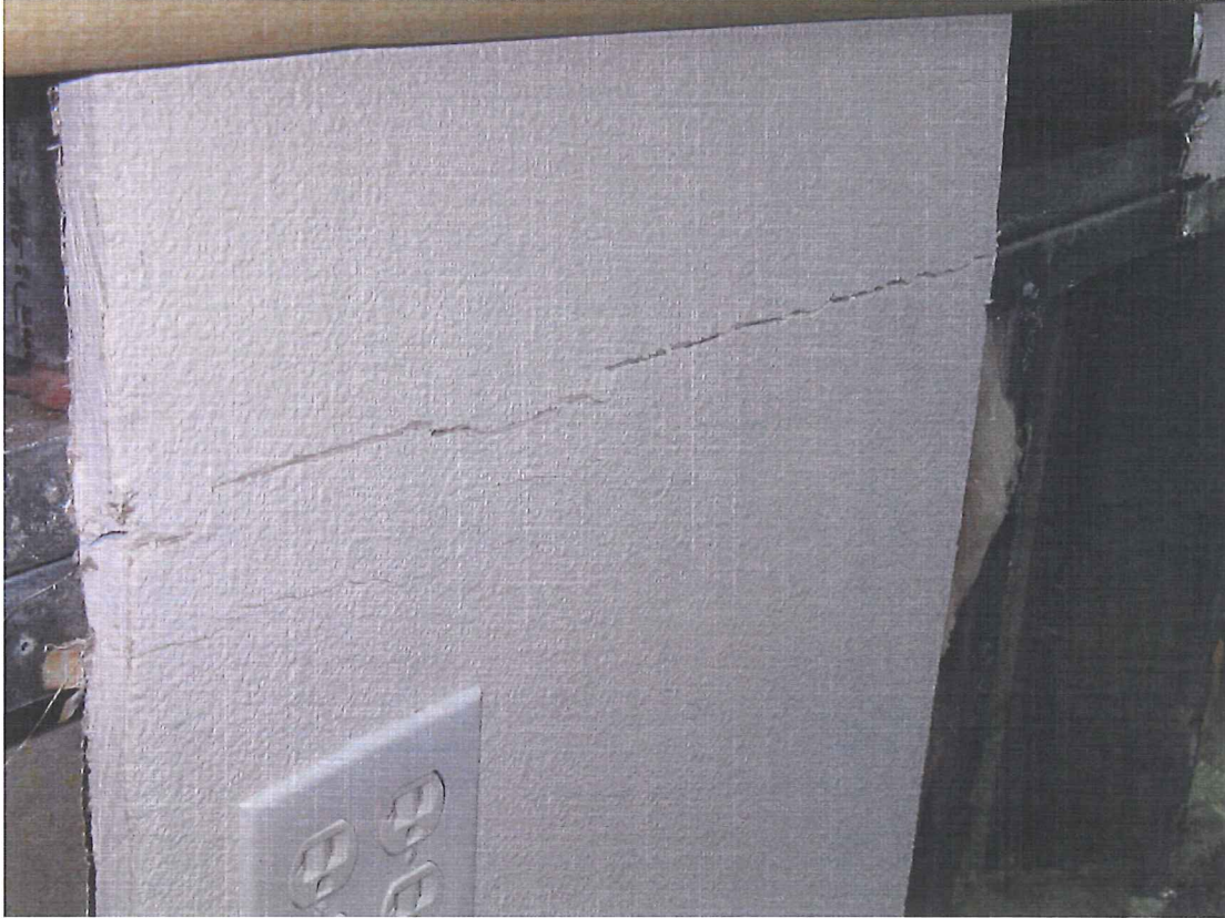
The framing at the horizontal crack is revealed Date: June 3, 2010
