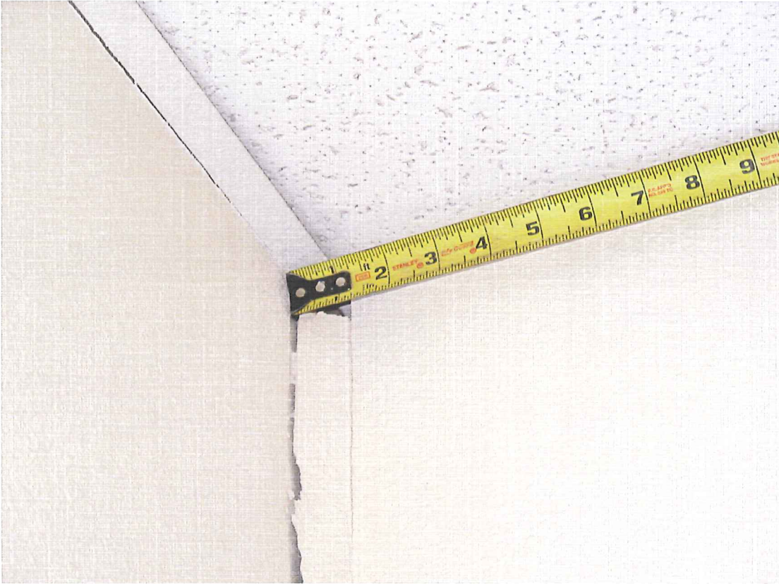
Interior partition walls pulling away from exterior wall with up to 1¼ inch movement measured on the fifth floor
