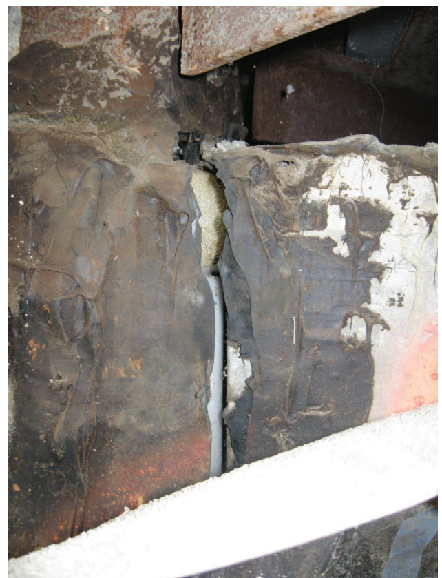
Bottom right: Joint between building and Bus Mall slab. Slab shortening ripped apart installed rubber water proofing.
