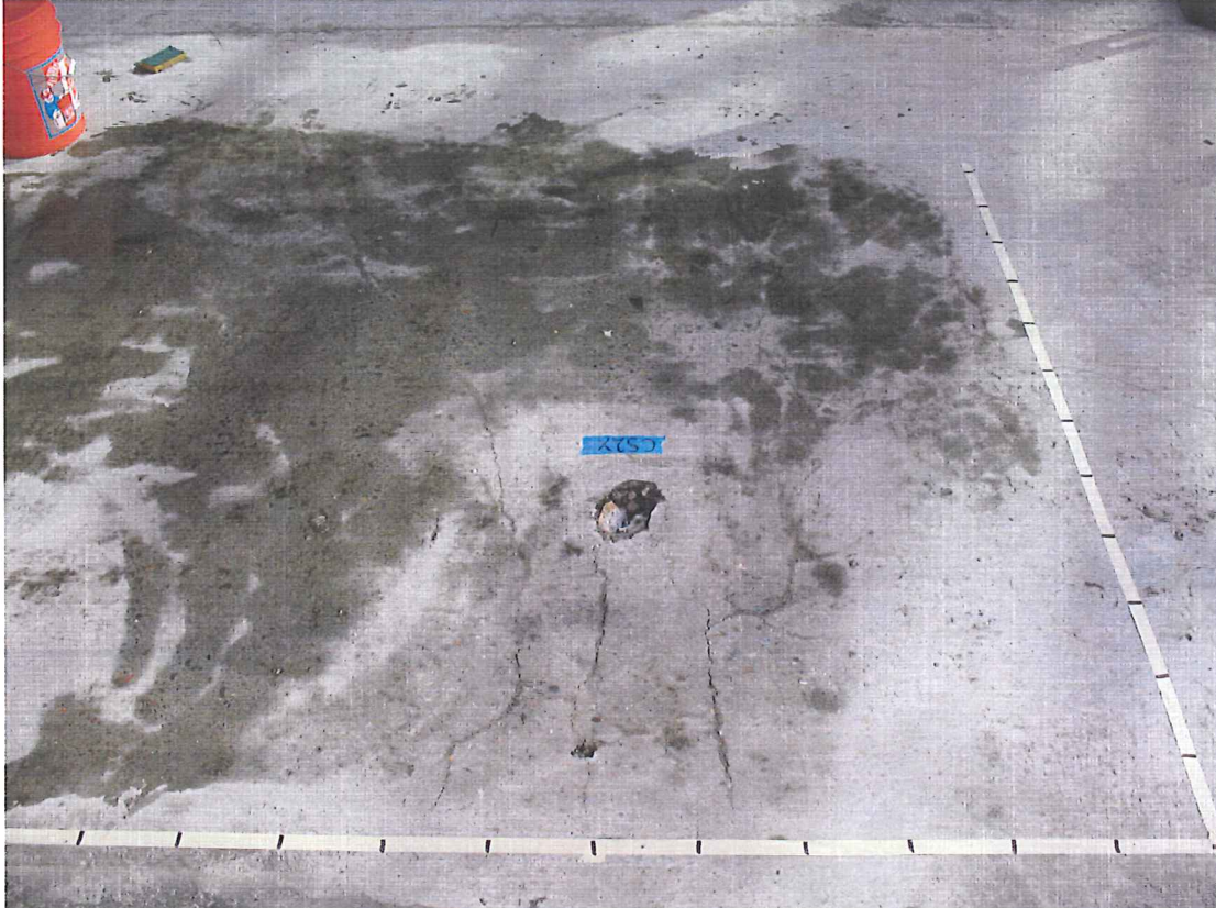
Bus Mall Punching Shear Location E-8 Date: June 30, 2010
