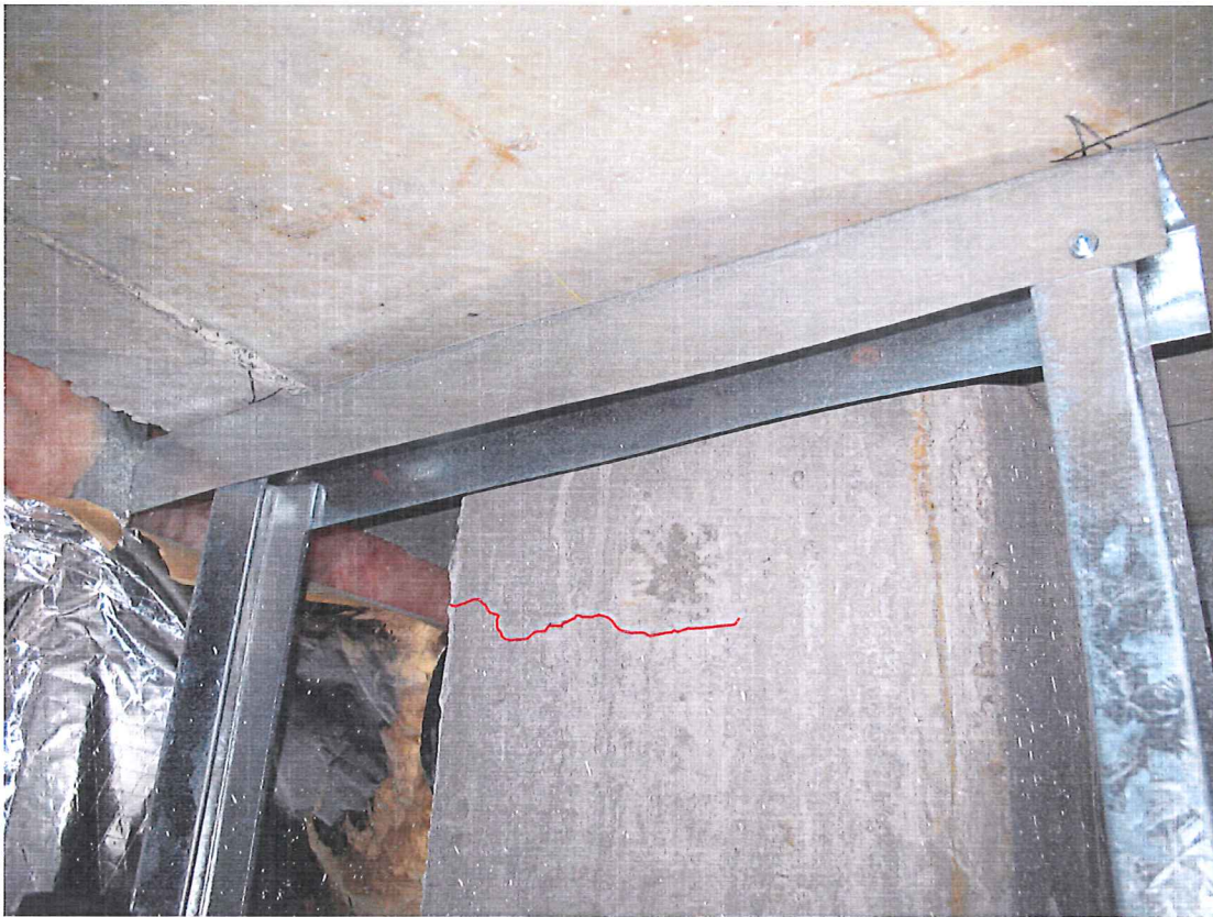
Cracking on outside face of column at the fifth floor Date: April 14, 2010
