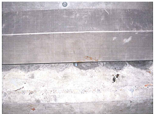
Close-up of grout pockets at Bus Mall Date: April 14, 2010
