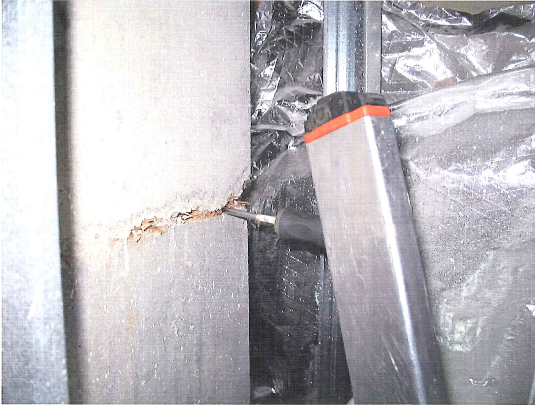
Screwdriver penetrating 2 inches into the concrete column Date: April 14, 2010
