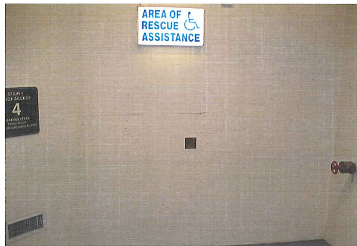
Horizontal cracking of concrete stairwells, Level 4, West stair tower Date: April 14, 2010
