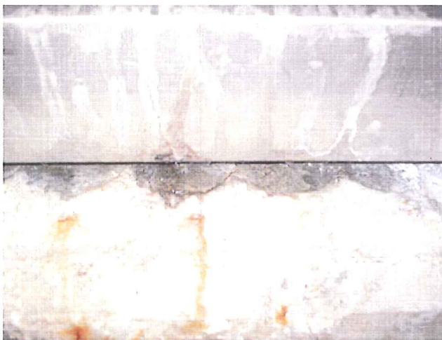
Close-up of grout pockets at Bus Mall Date: April 14, 2010
