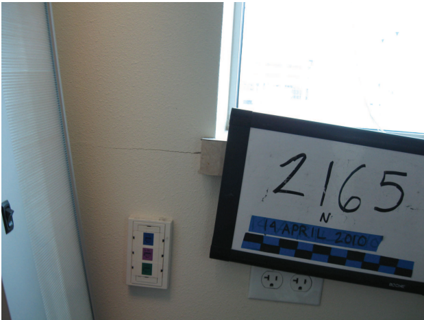
Top left: Wall crack with repair attempt.
