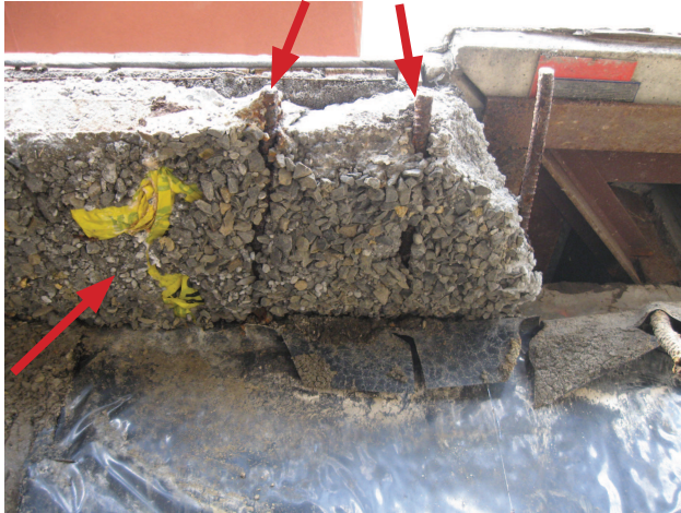
Top left and right: Reinforcing bars not installed properly. Debris is evident in the casting bed during construction.
