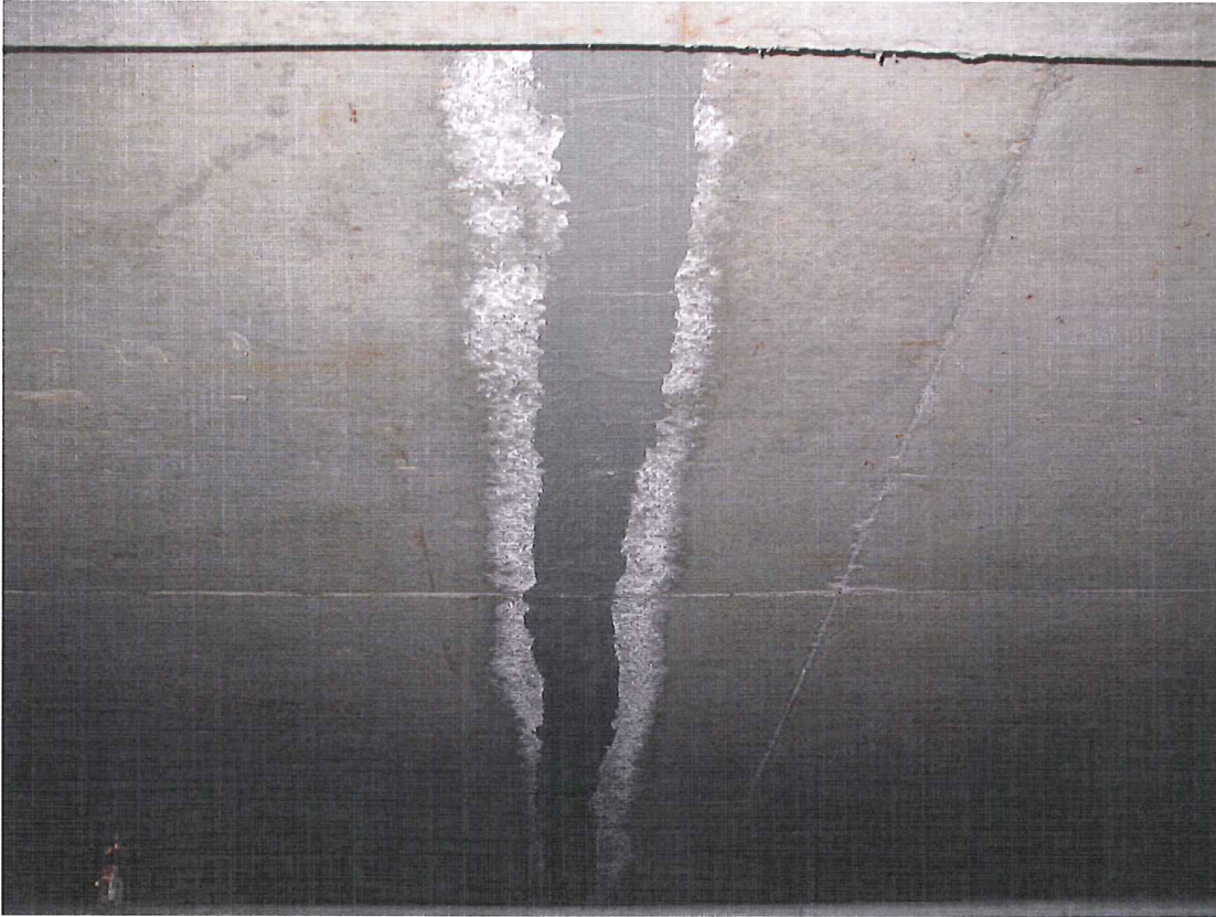
Cracking at midspan between columns as a result of thermal expansion of the exposed PT slab Date: April 14, 2010
