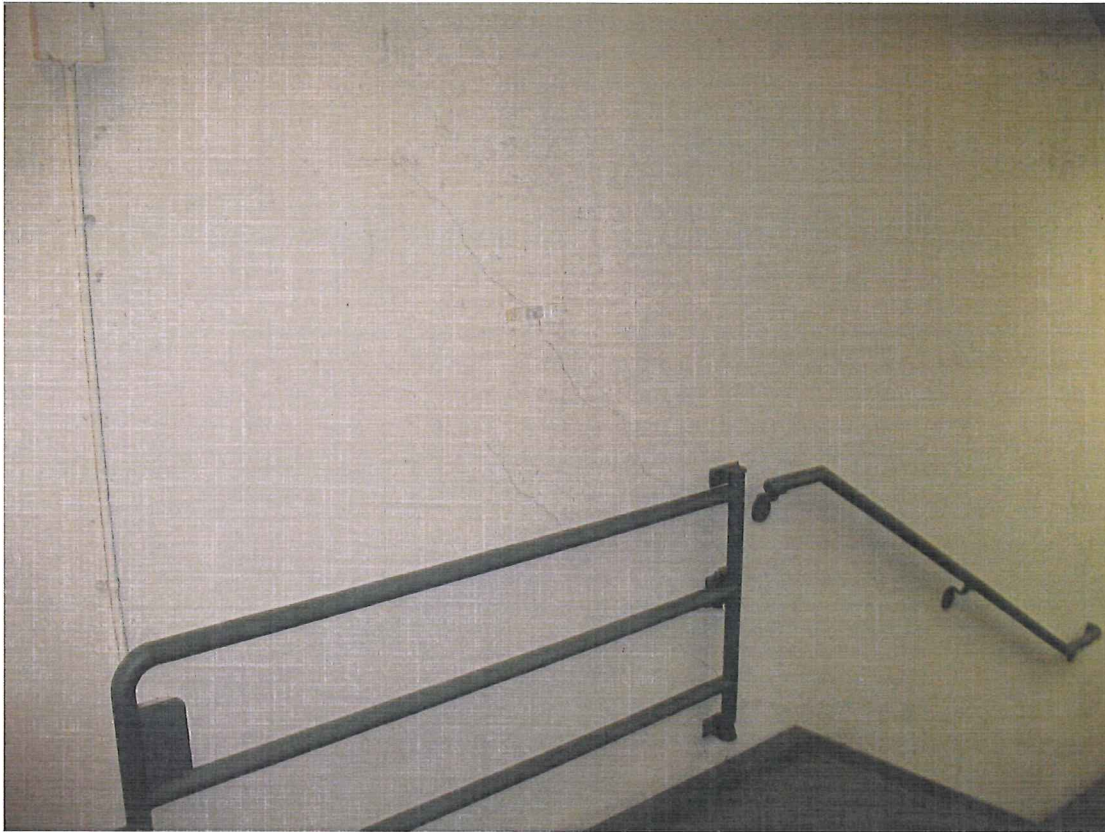
Several diagonal cracks on the ground floor on the north wall of the west stair tower Date: April 14, 2010
