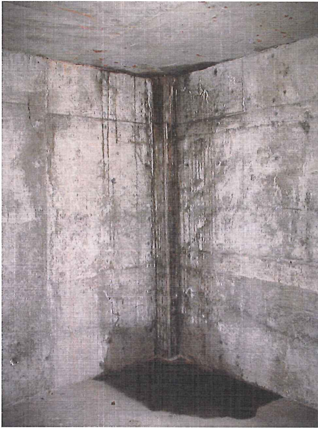
Significant cracking and efflorescence coming through concrete at Northeast corner column (Grid N1-1) Date: December 1, 2010
