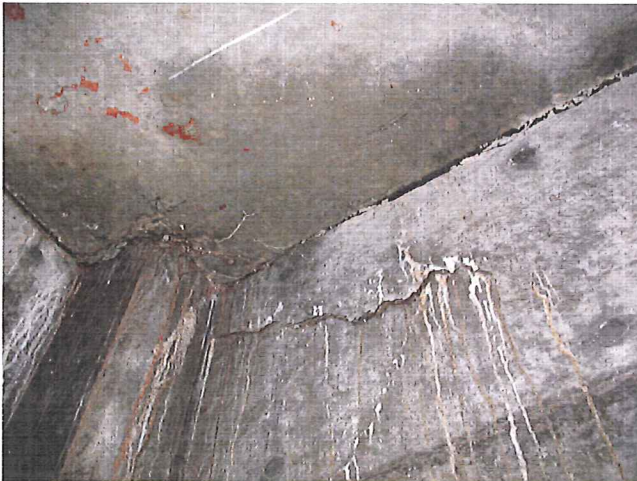
Significant cracking and efflorescence coming through concrete at Northeast corner column (Grid N1-1) Date: December 1, 2010
