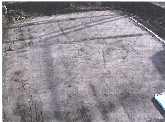
Bus Mall Punching Shear Location C-5 Date: June 30, 2010
