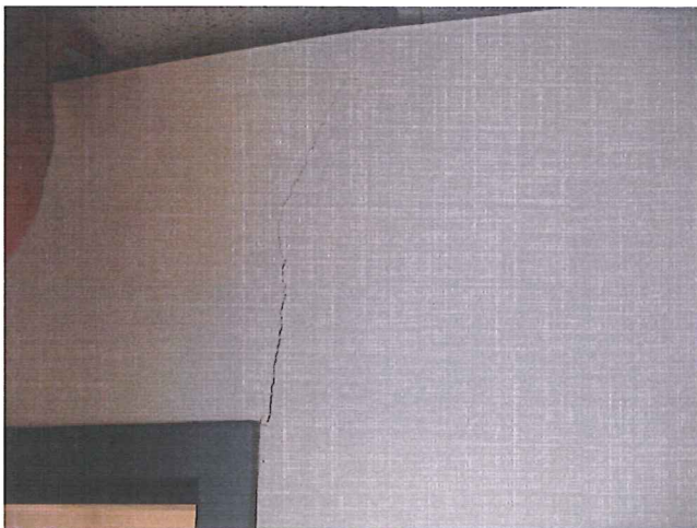
Racking of door frames and cracking of the wall finish Date: April 14, 2010
