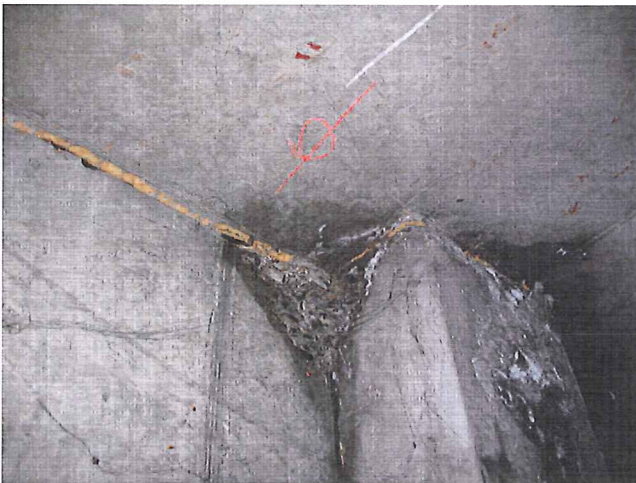
Significant cracking and efflorescence coming through Concrete column at Grid M-1 Date: December 1, 2010
