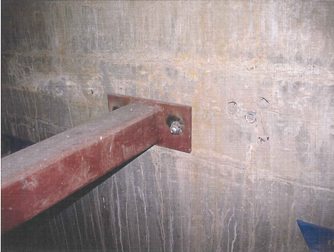
Elevator Hoistway – Stabilizing bar installation at floor slab (excess drop-in anchors visible to the left) Date: April 14, 2010
