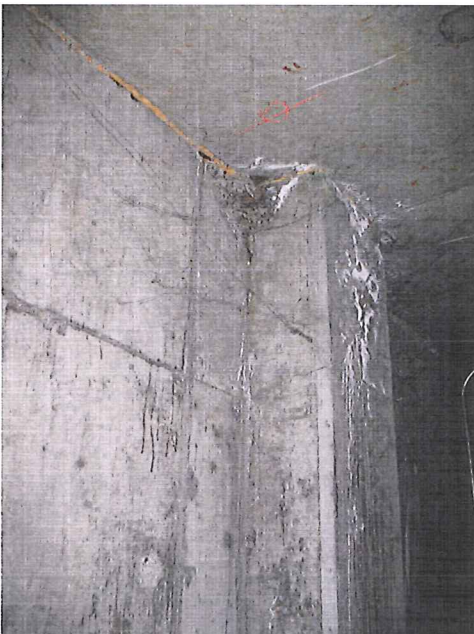
Significant cracking and efflorescence coming through concrete column at Grid M-1 Date: April 14, 2010
