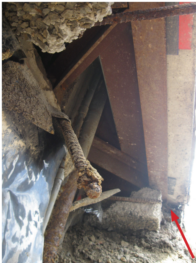
Bottom left: Installed reinforcing bar bent during construction was not repaired. Bar in background indicated proper installation depth.
