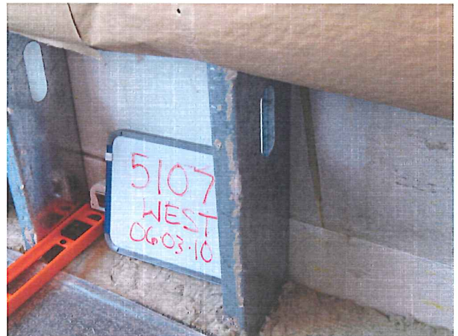
Twisting of the exterior structural light gauge steel studs Date: June 3, 2010
