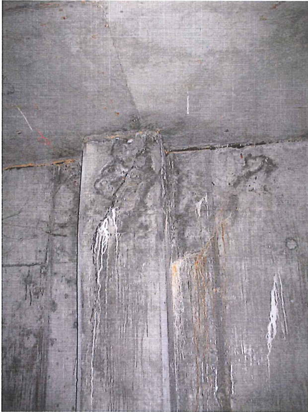
Significant cracking and efflorescence coming through Concrete column at Grid M-1 Date: January 5, 2011
