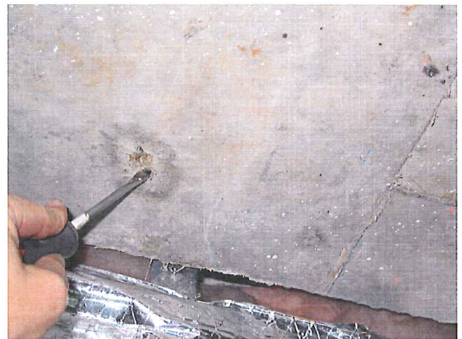
Debris inside slab Date: April 14, 2010
