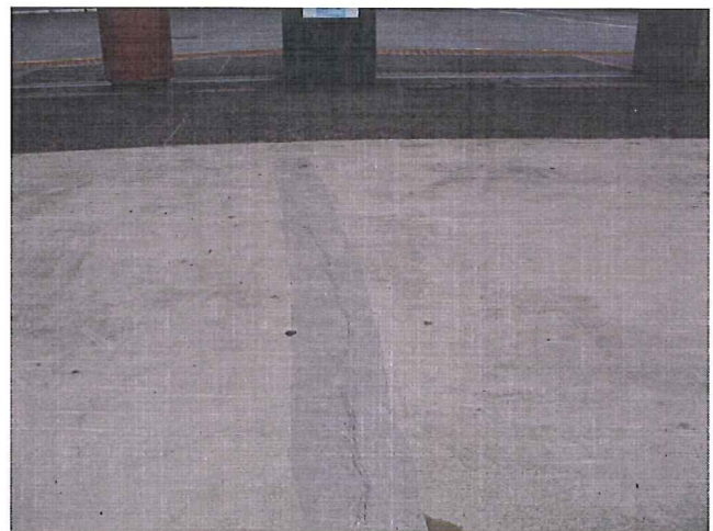
Jointed repair at the top of the PT slab Date: June 1, 2010
