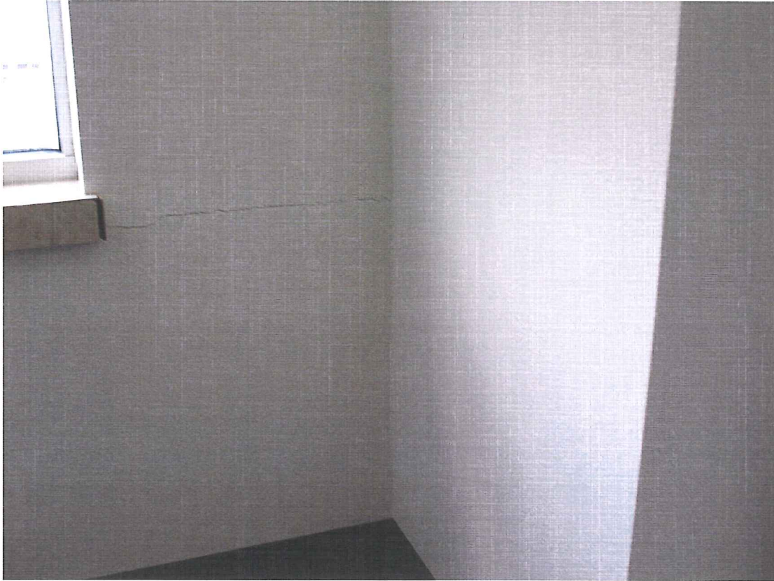
Horizontal crack at the base of the windows, which was observed on the third, fourth and fifth floors. Date: April 14, 2010
